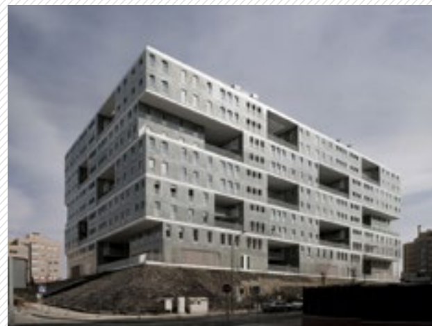
Celosia building, Madrid, MVRDV
